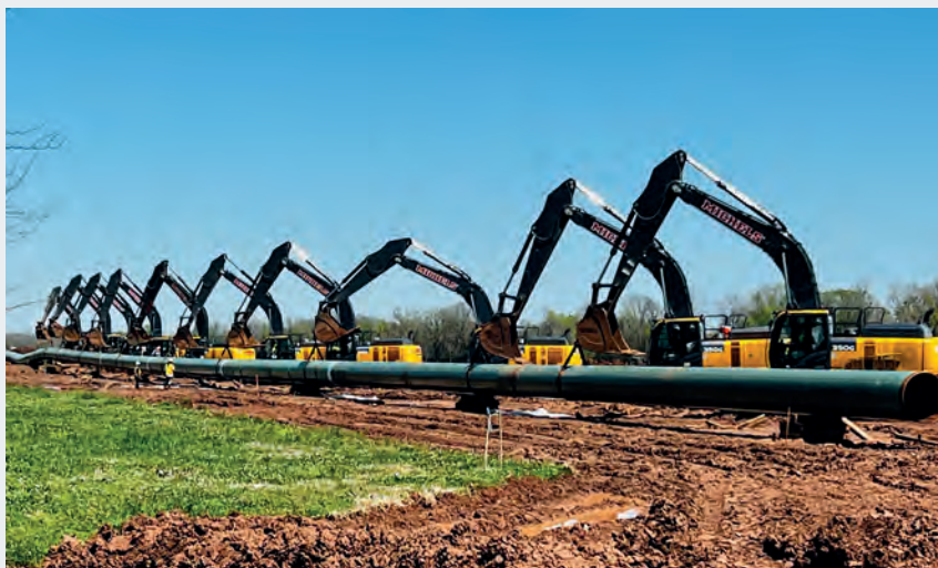
Figure 1. Michels Pipeline constructed 134 miles of 42 in. pipeline to deliver natural gas from supply basins in the Haynesville shale play in northeast Louisiana to liquid natural gas terminals along the Gulf Coast.
