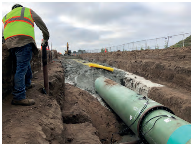
Figure 3. Carrier pipeline and casing prior to backfill, with lead wires routed to test station conduit.
