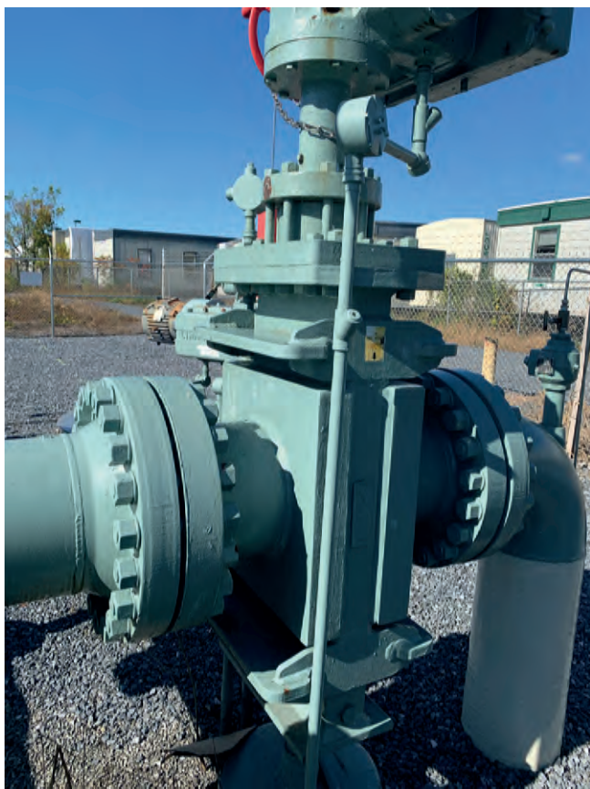
Figure 2. Replacing the valve seat, gate, and stem every 10 years as a precaution is good practice.
