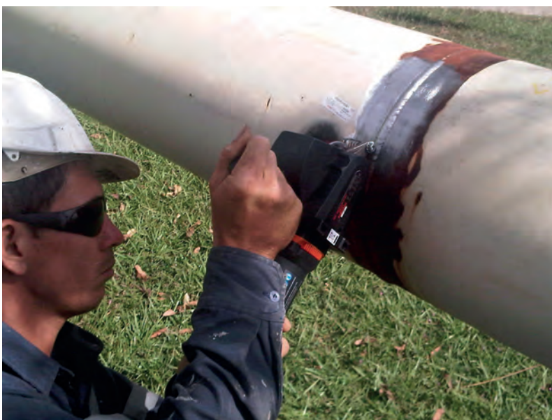
Figure 3. Bristle blasting a field joint.
