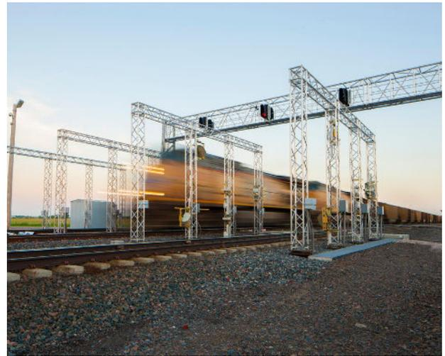
*Machine visioning can take 1,000 images per rail car at speeds up to 70 mph, identifying defects early for maintenance.*
