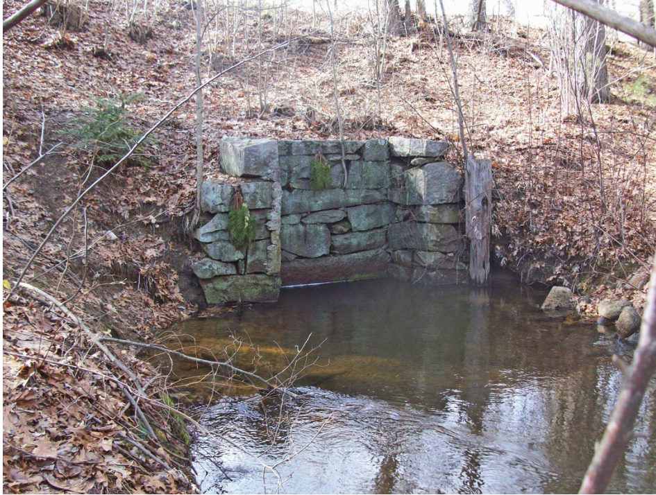
Stone work at the Archbrook Culvert (photo by Steve Klomps, 2017)
