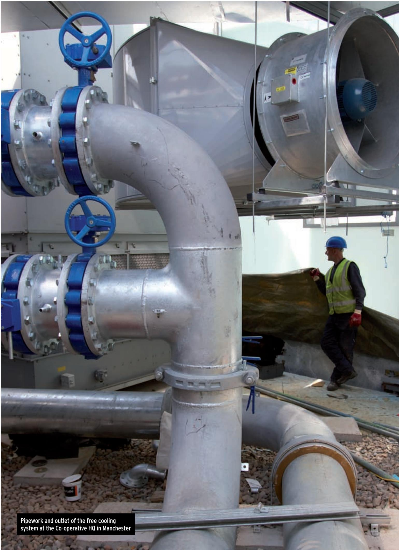
Pipework and outlet of the free cooling system at the Co-operative HQ in Manchester
