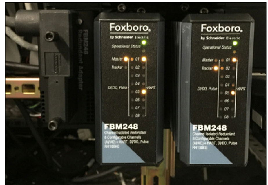
With the Foxboro Evo FBM248, Schneider Electric introduced redundancy capabilities to its Intelligent Marshalling, its form of universal I/O.
